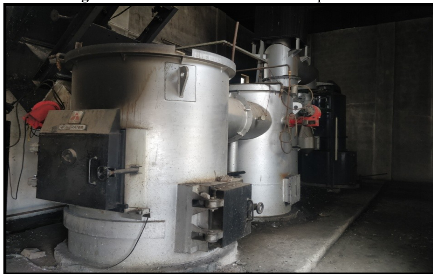
Figure 3: The incinerator at district hospital Leh
